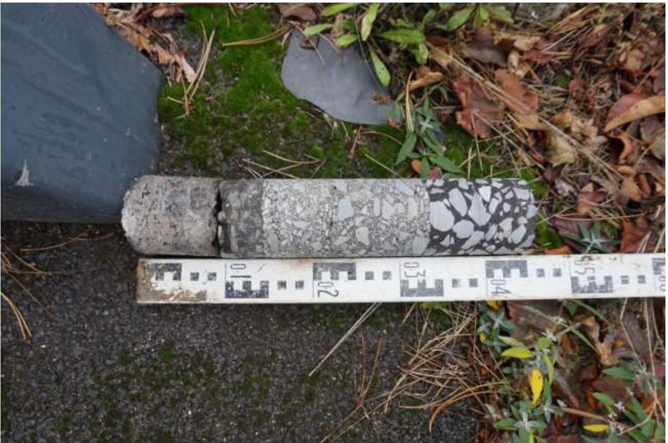
Plate 28: 0.45m high core sample extracted next to the main gate showing great depth of road layers
