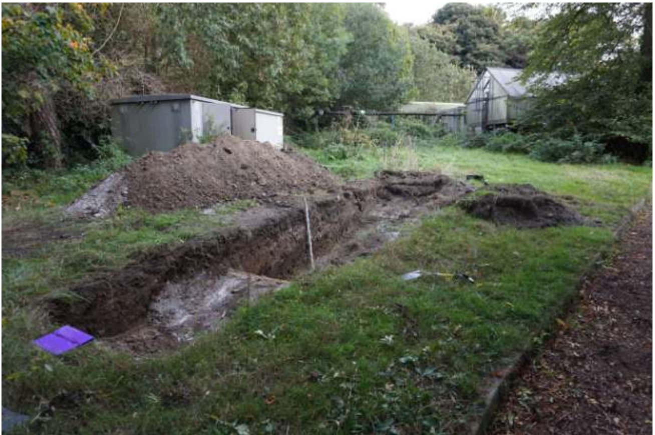
Plate 21: Looking east at Trench 9
