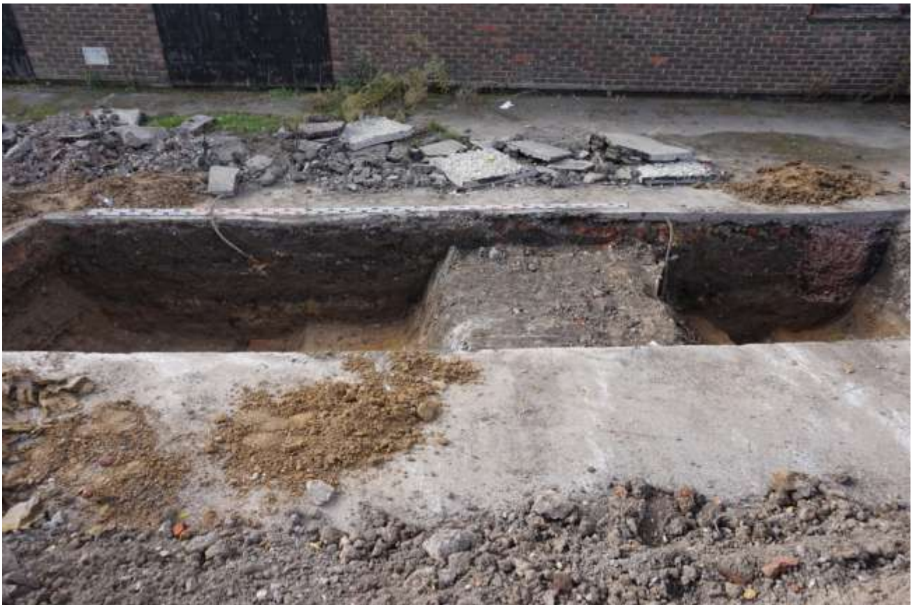
Plate 12: Looking south west at section of Trench through modern deposits overlaying modern ditches
