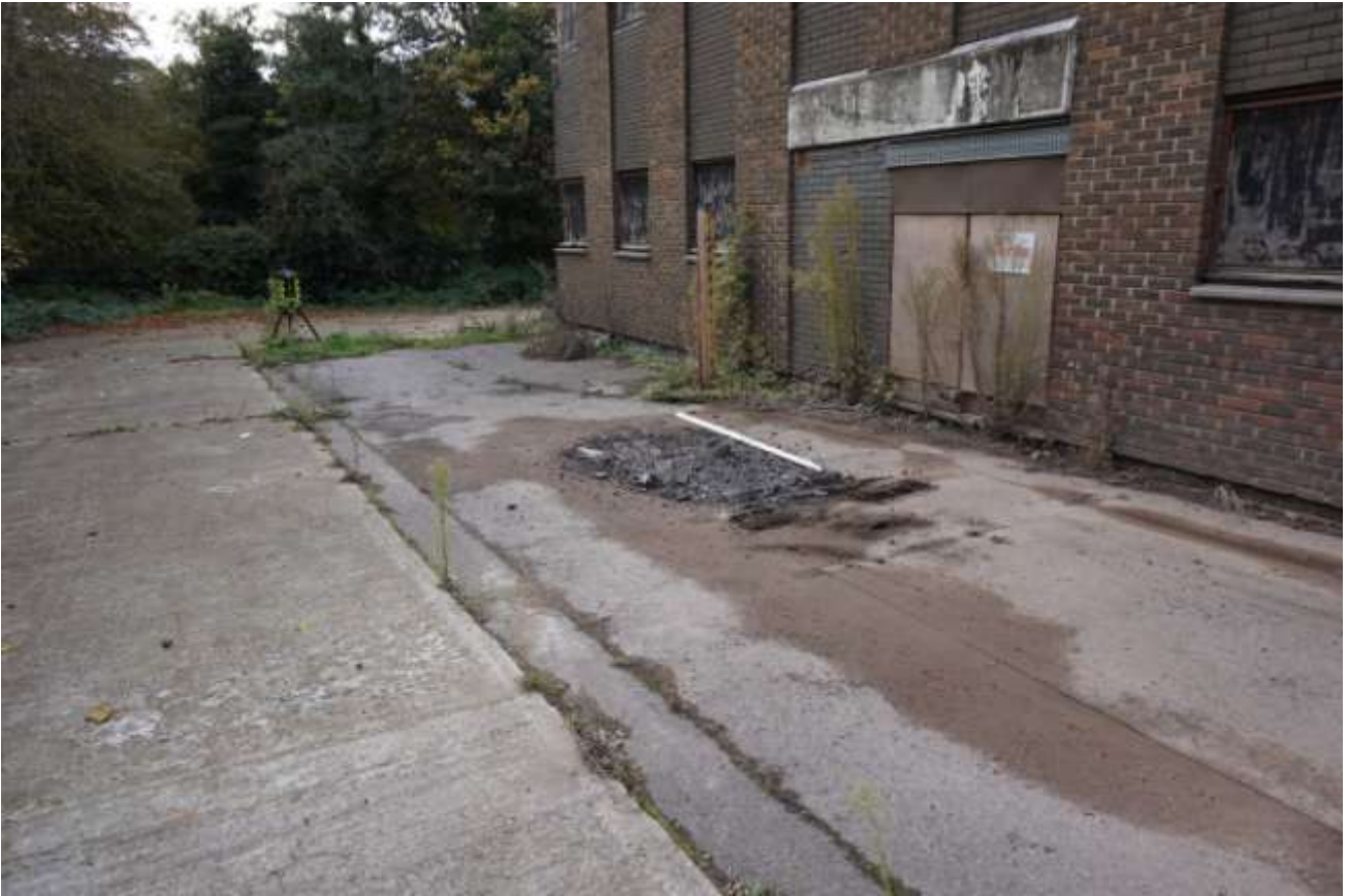
Plate 18: Looking west at attempt of excavation of Trench 6. Underneath tarmac layer concrete has been exposed.
