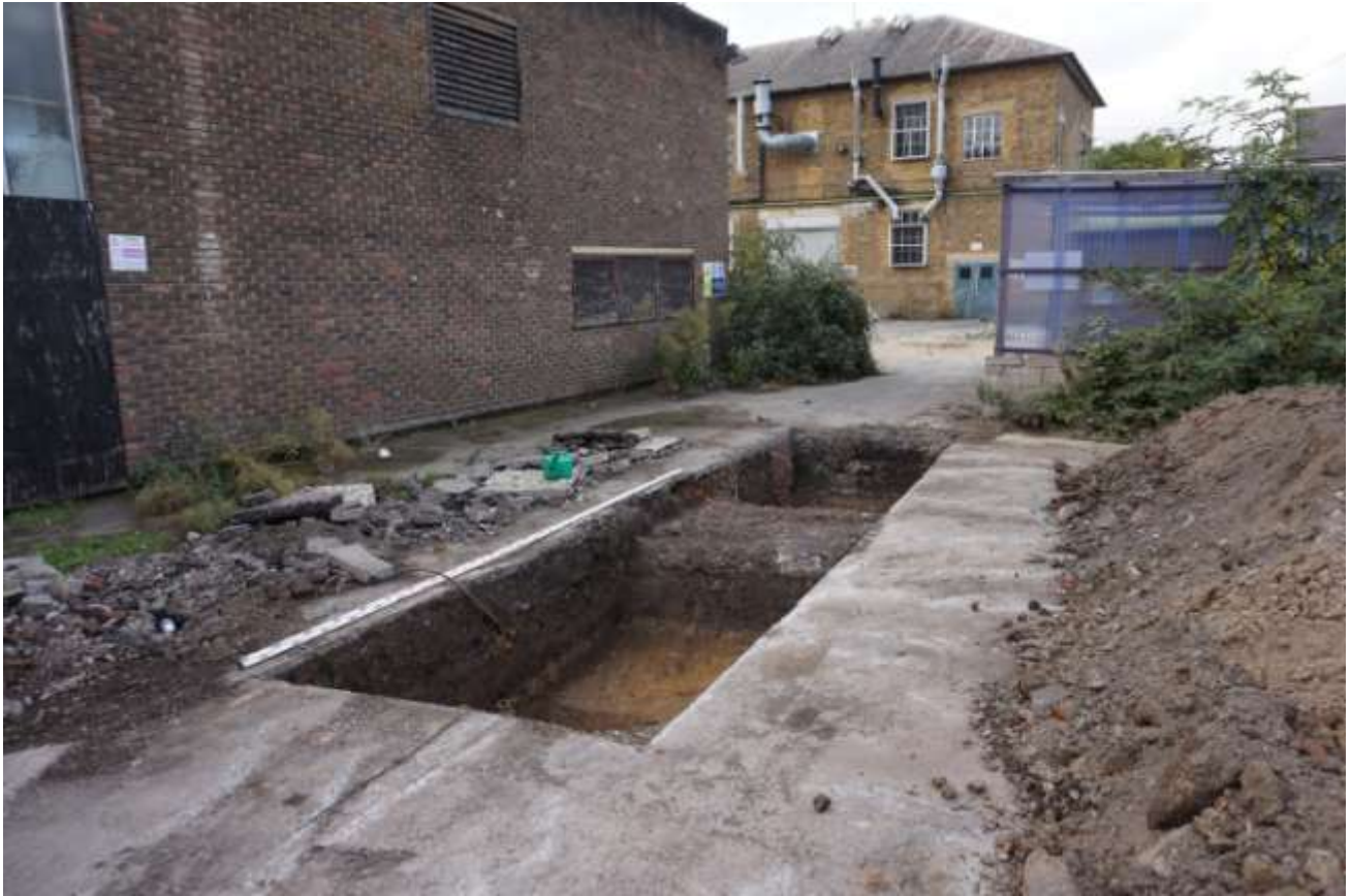
Plate 11: Looking north west at Trench 5; five metre scale.
