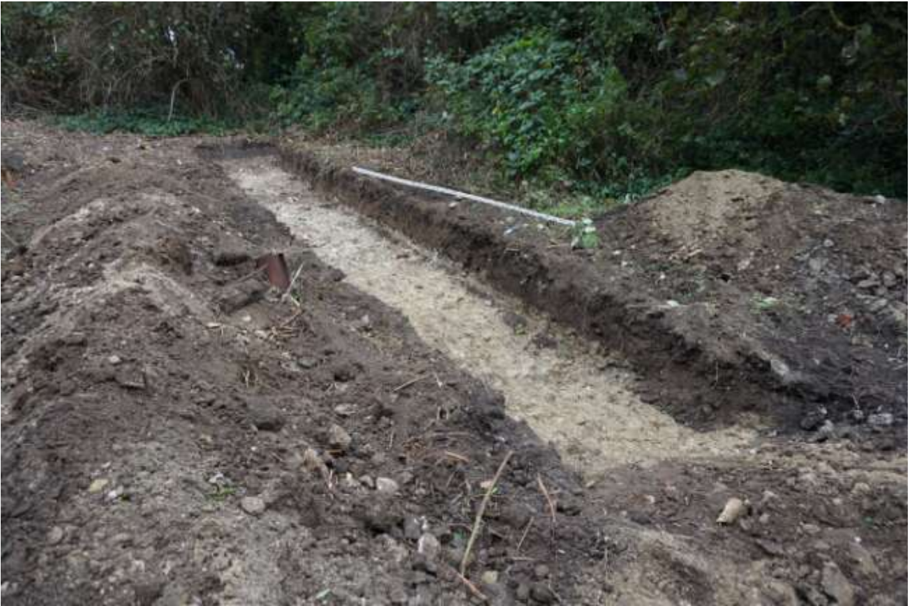
Plate 25: Looking east at Trench 12
